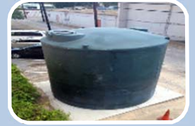
City of Weslaco Rain Harvesting System Weslaco Library LID Project
