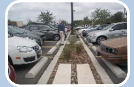
South Texas College Biofilter/Bioretention System, McAllen, TX
