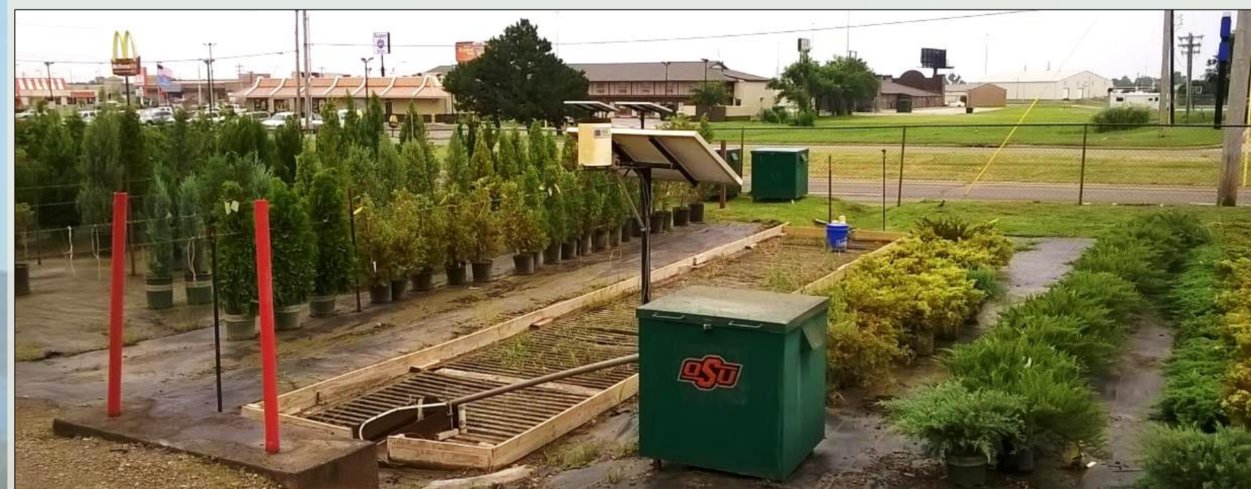
Figure 5 – Project site, sampler set up for inflow, wooden barrier surrounding cell.
