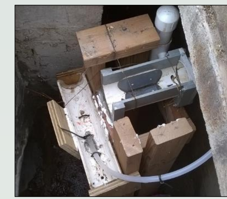
Figure 4 – Underdrain flow measurement
