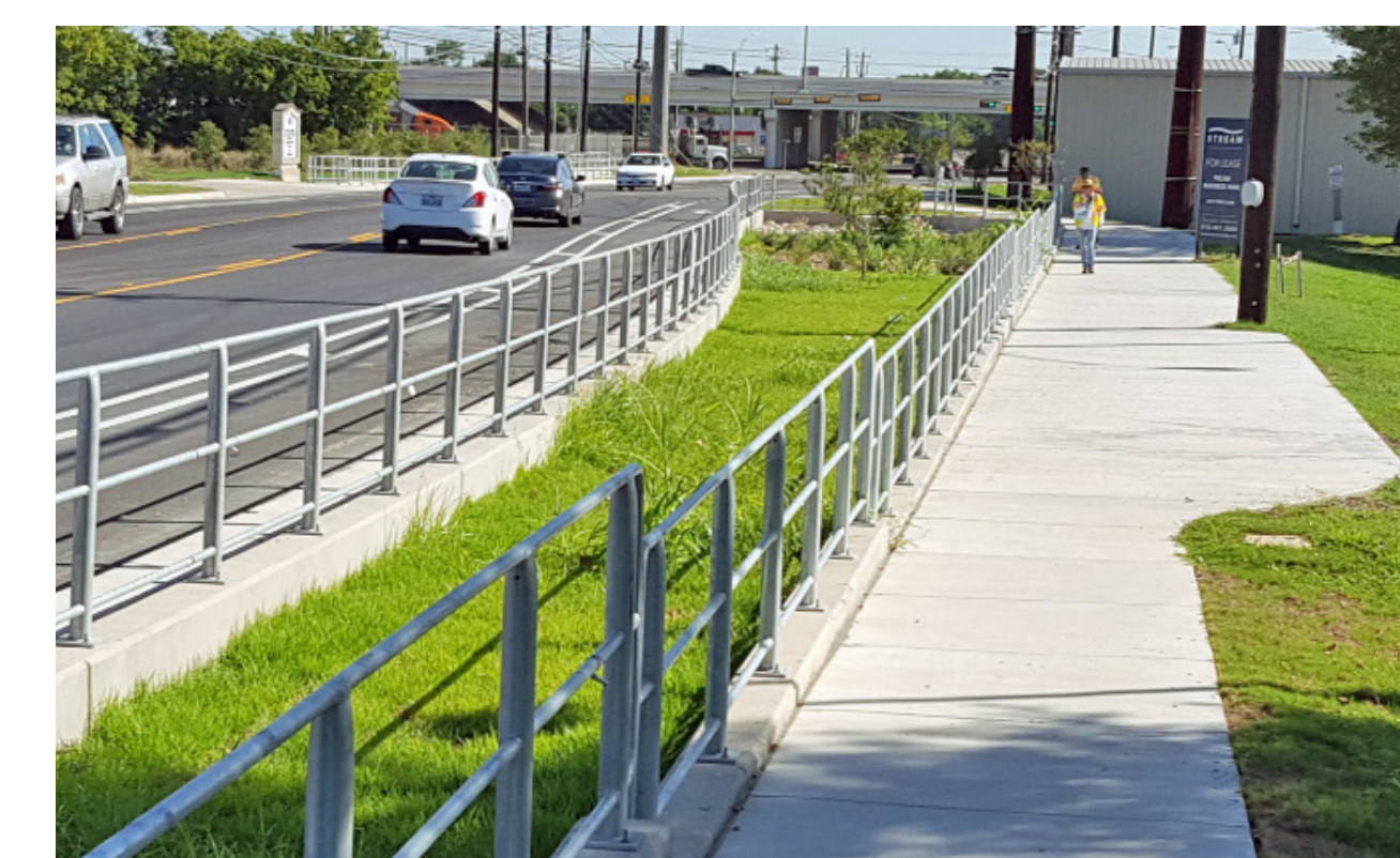
Rain Garden 2: Sidewalk expands from 6 - 10 feet to allow vehicular access for maintenance.
