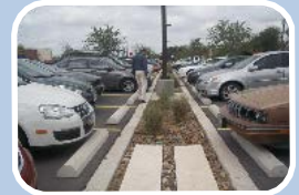
South Texas College Biofilter/Bioretention System, McAllen, TX
