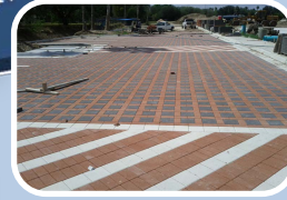
City of La Feria Recreational Center LID Pervious Paver Project
