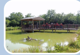
Constructed Wetlands Valley Nature Center Weslaco, TX
