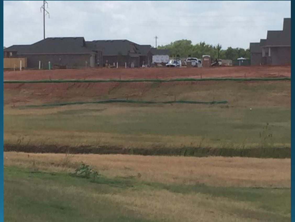
Filtrex in place of silt fence for perimeter control
