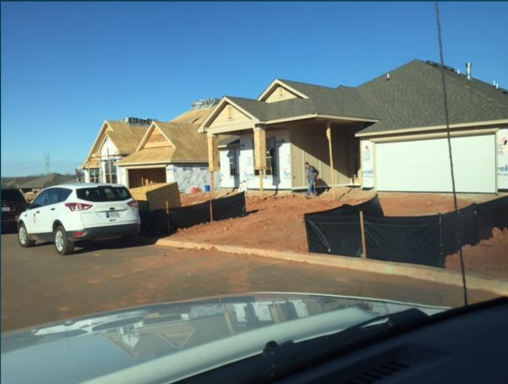
Silt Fence installed day one:
