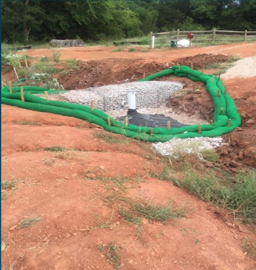
Filtrex stacked to protect project
