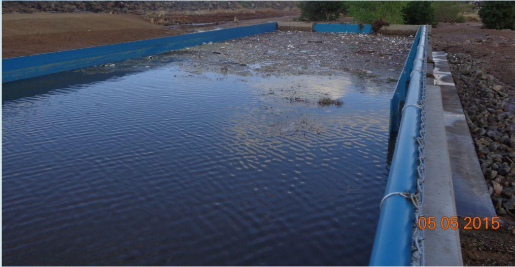
Stormwater detention pond with floatables baffle
