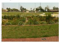
Bentley Athletic Park in Bixty, Oklahoma, is home to a rain garden in the middle of a new roundabout. Water drains into the rain garden through pipes from the surrounding athletic fields and soaks into the ground. Exess water enters the storm sewer system through a riser within the rain garden.
