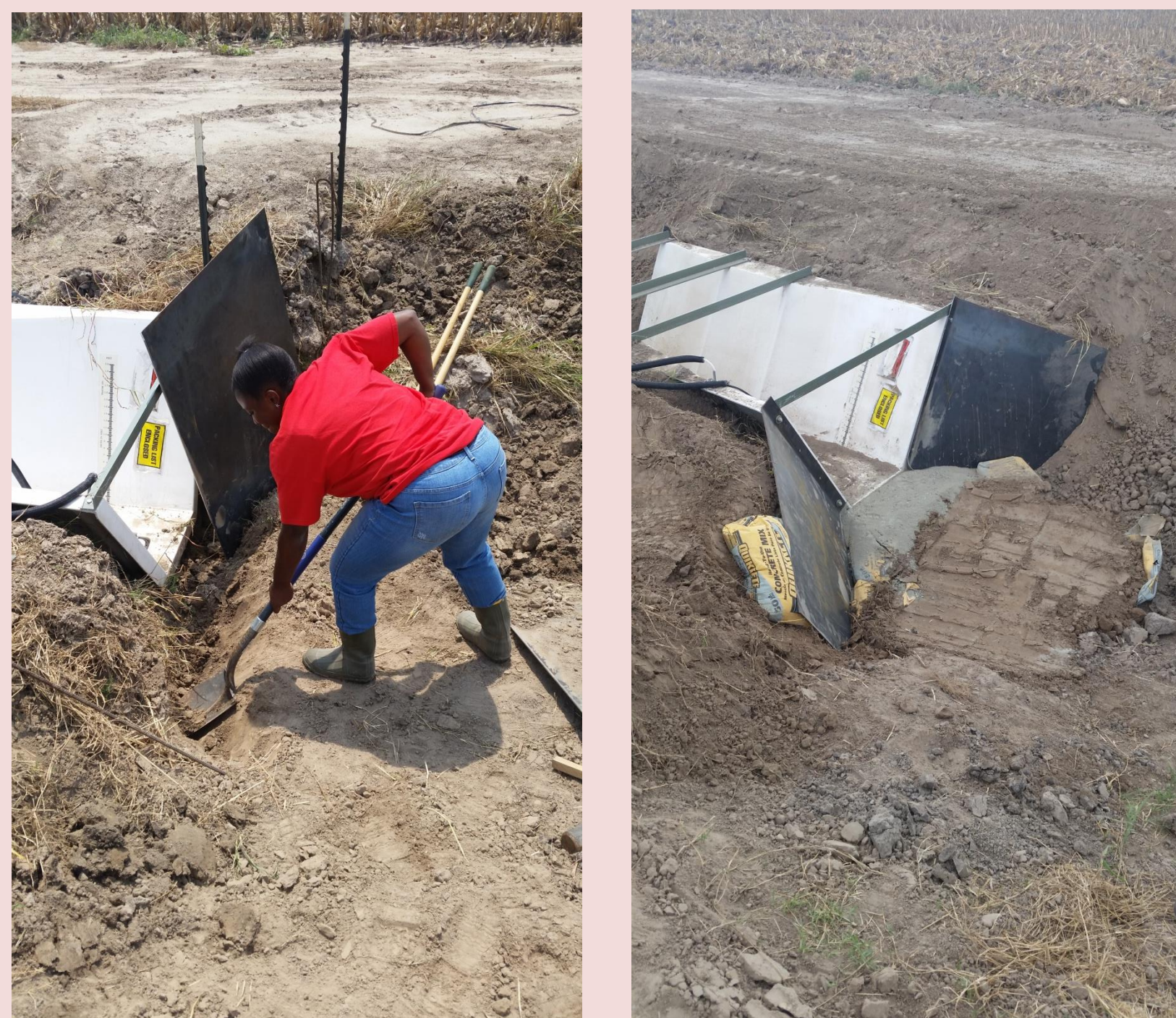
Fig. 3 Lonoke County Site 2: Site has no open-channel pipe present. Runoff volume will be calculated from pressure transducer measurements and water depth with the appropriate equations for use with the trapezoidal weir.
