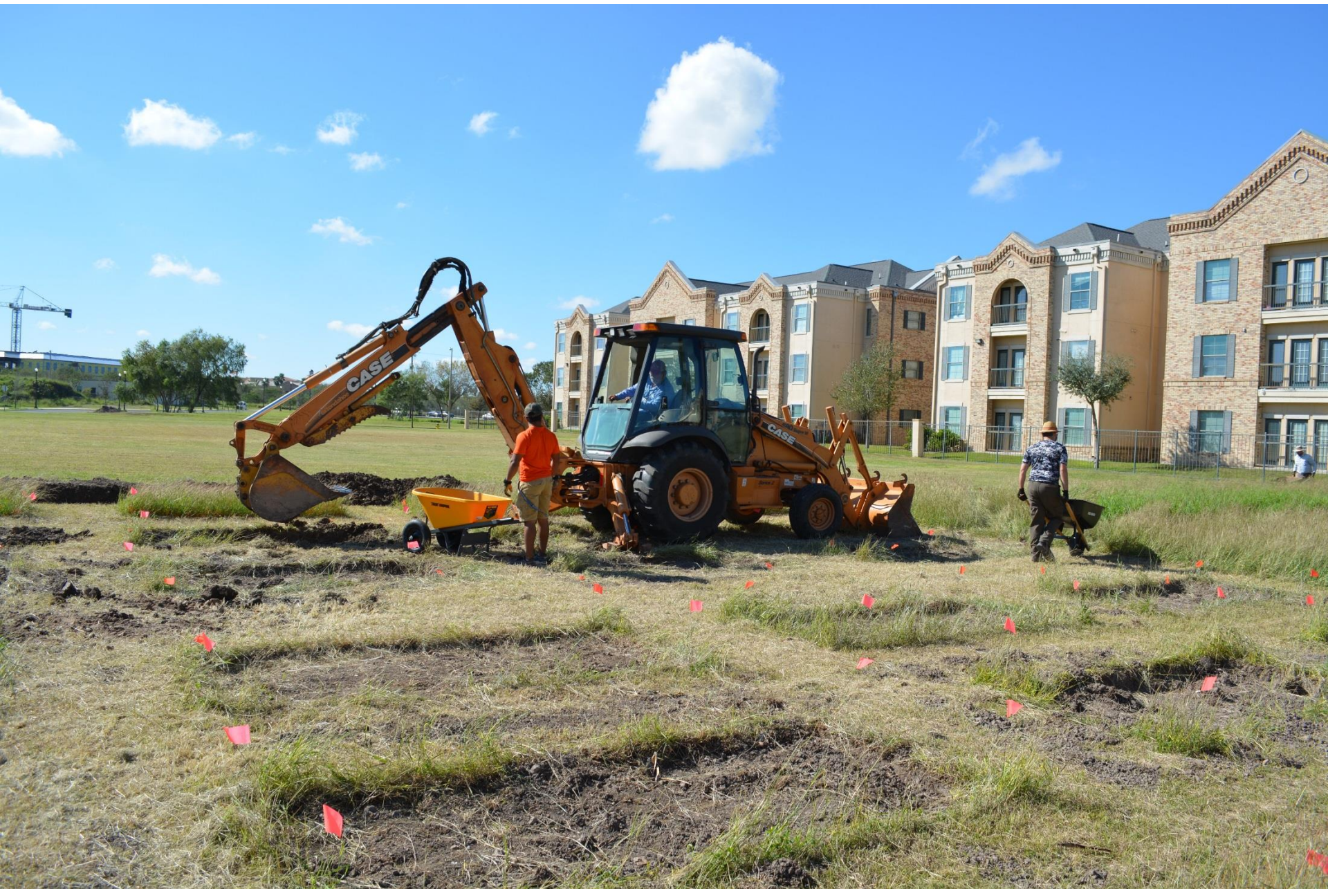
Jan 2017 – Campus Facilities Operations donated a backhoe and operator time.
