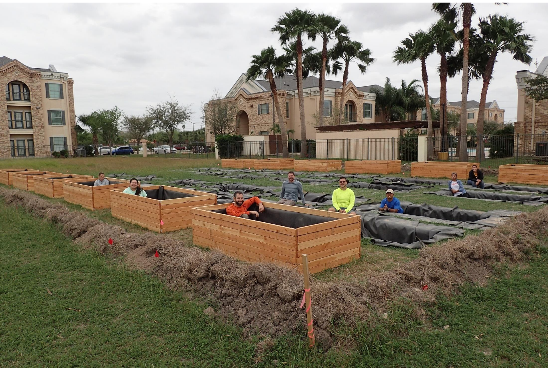
Feb 2017 – Construction complete. Next step: move 60 cubic yards of soil (4 dump trucks).
