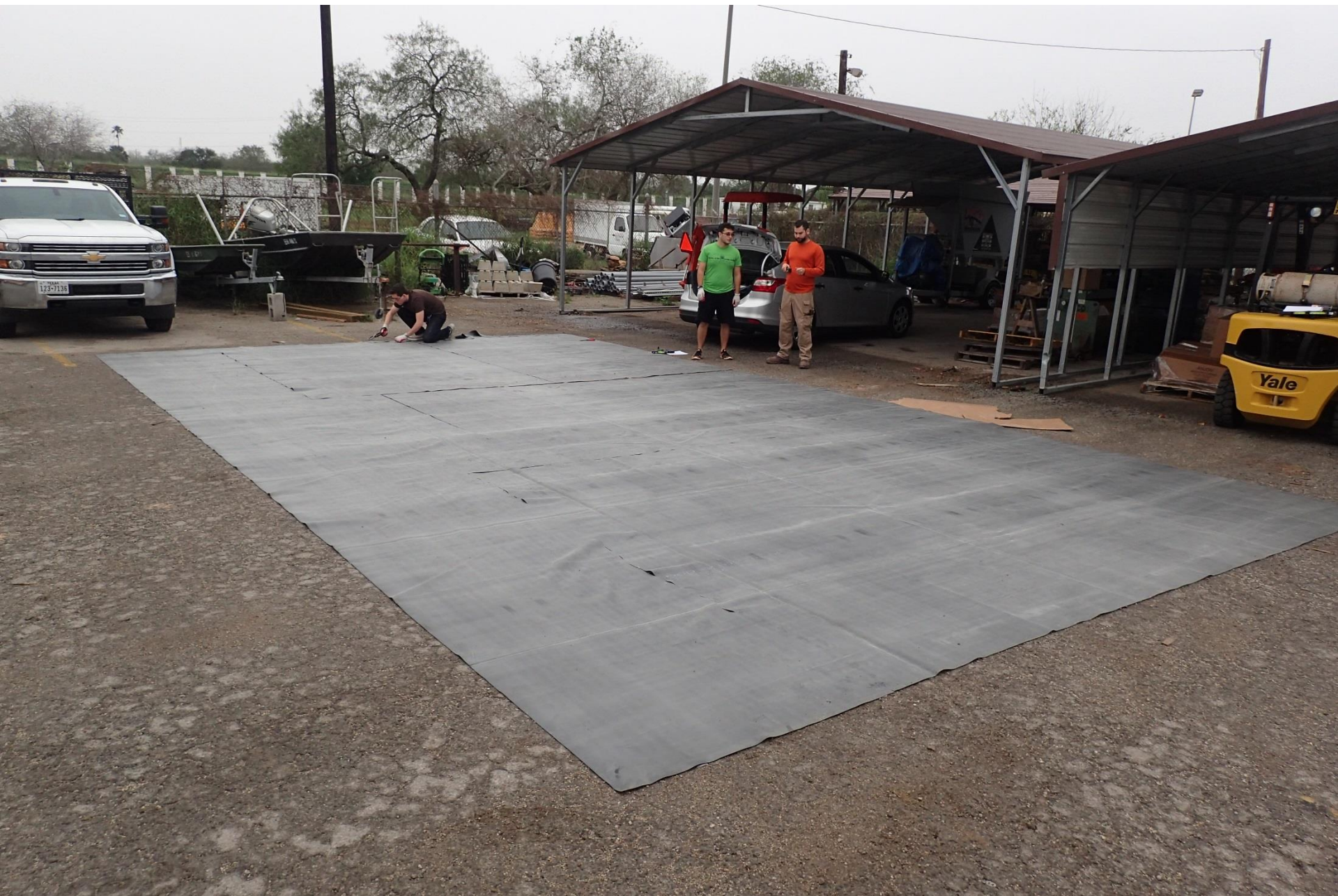
Jan 2017 – Plumbing began by cutting 60 mil rubber liners to size; each roll weighed 180 lbs.
