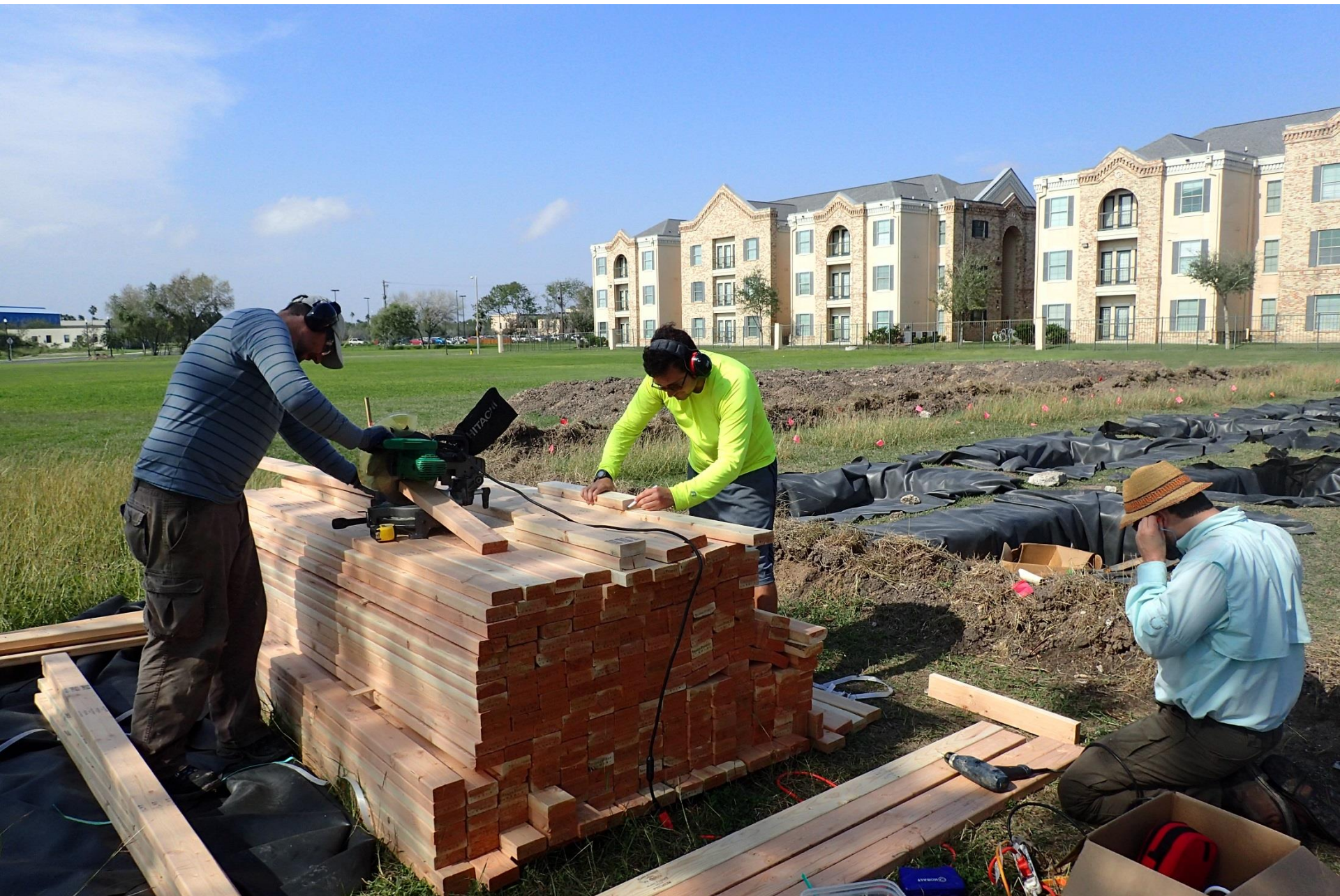
Feb 2017 – With wetlands and ponds lined, we began building the raised beds.
