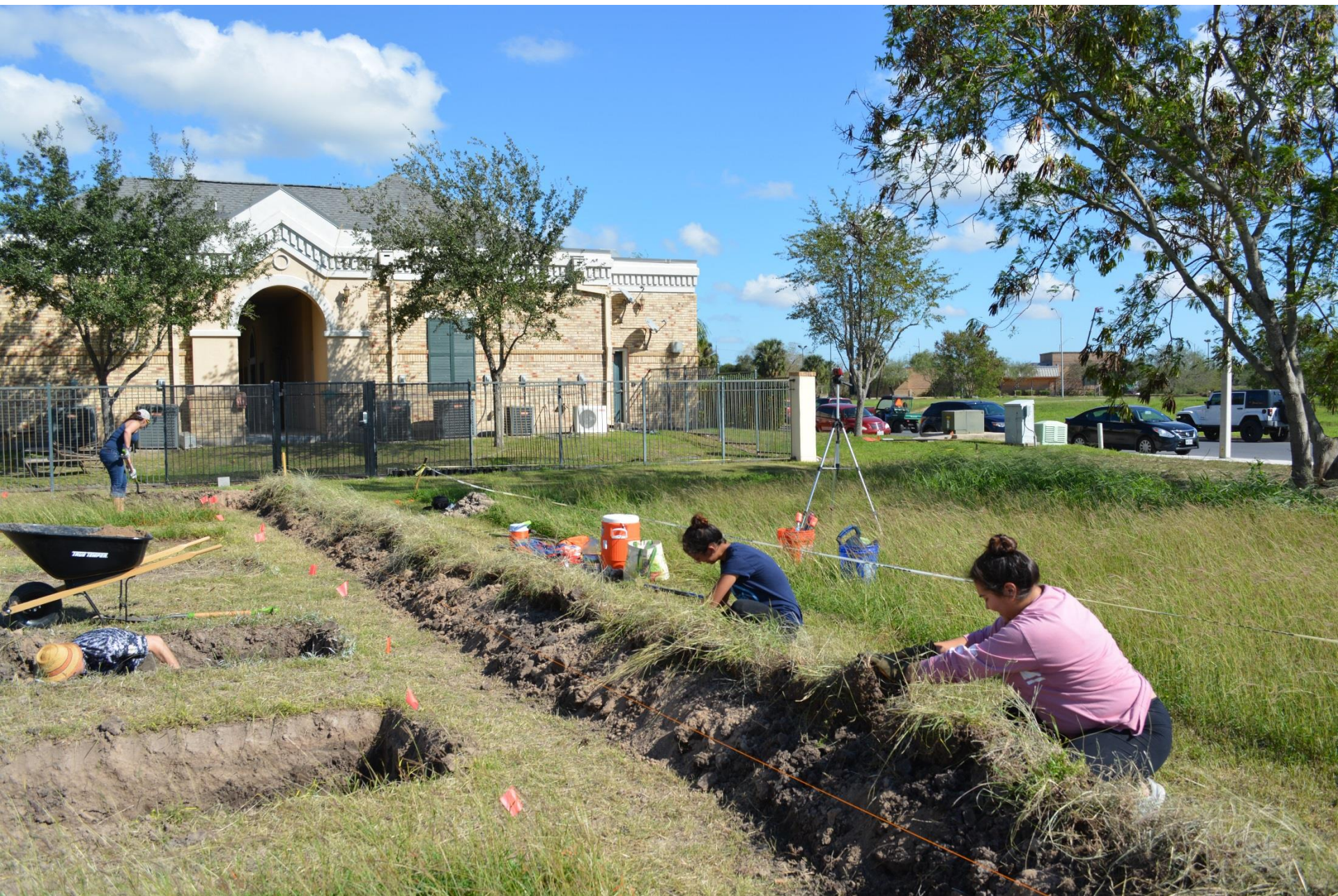
Jan 2017 – Students shape the earthen berm and arrange sod to reduce erosion.
