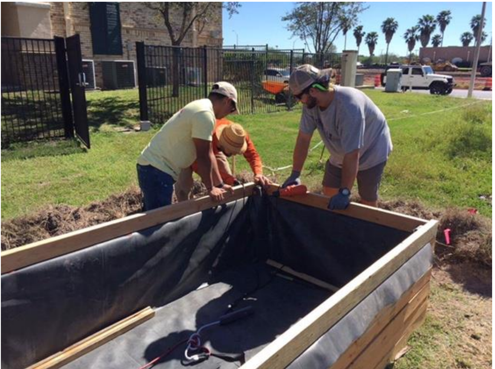
Feb 2017 – Raised beds were lined with rubber to capture water and move it to wetlands.
