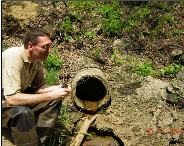
Figure 12: Dry weather field inspection
