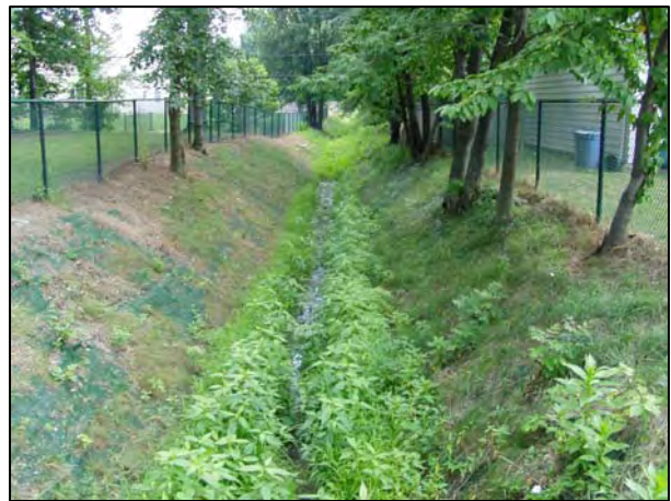
Figure 3: Ditch MS4 outfall
