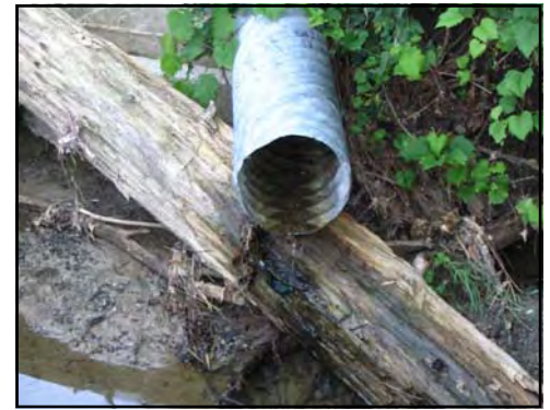
Corrugated Metal Pipe (CMP)
