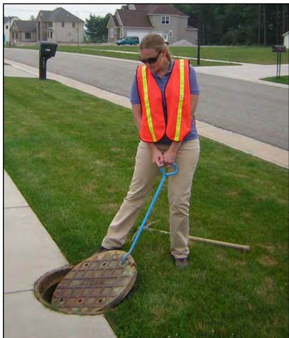
Figure 14: Removing storm drain lid
