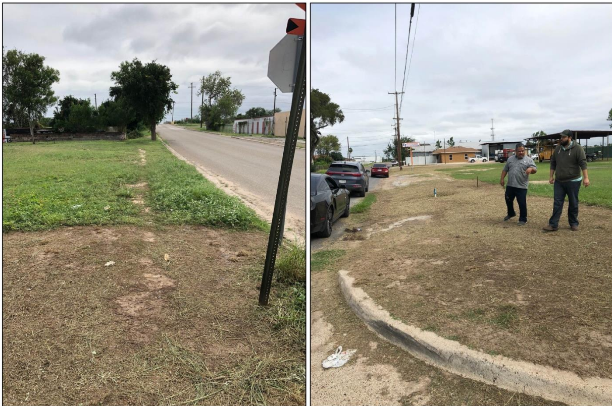
Figure 18. Site selected for the permeable pavement before construction
