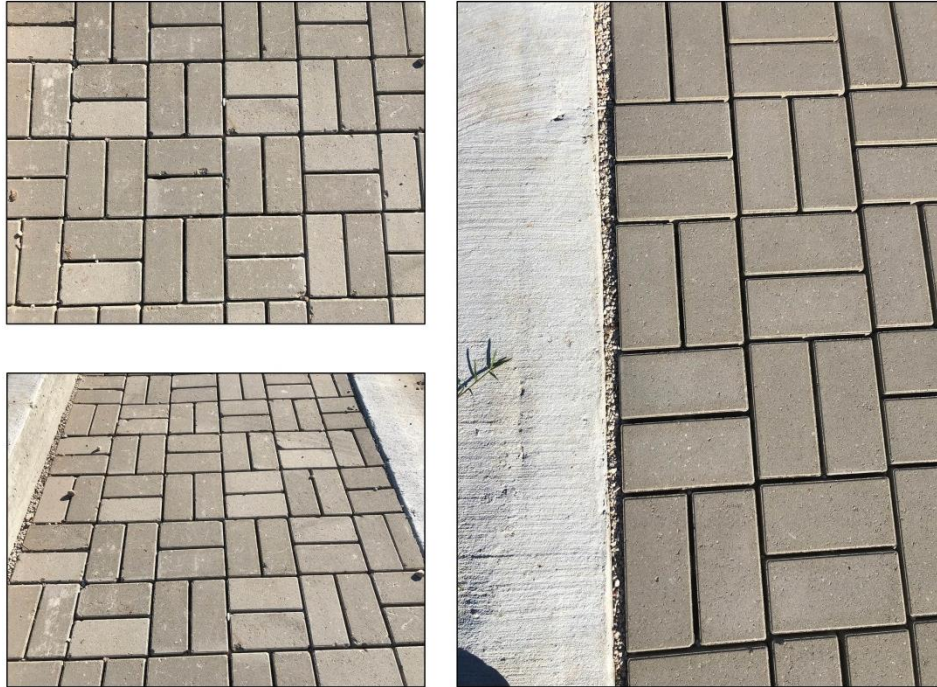
Figure 21. The permeable pavement joints filled with gravel to increase the runoff infiltration
