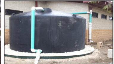
Rain Harvesting system (Weslaco, TX)
