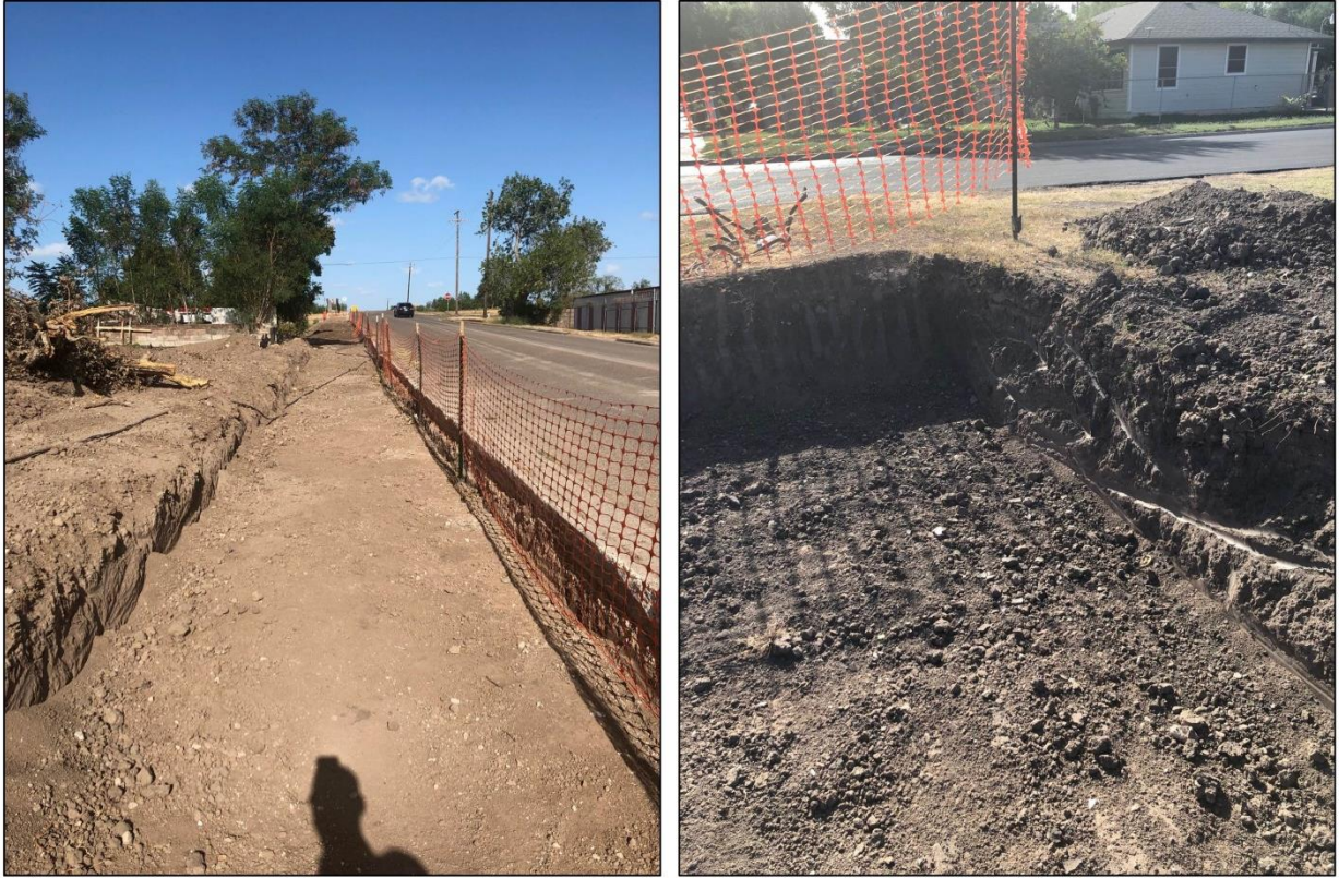
Figure 19. Construction of the permeable pavement
