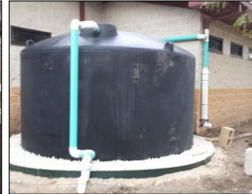
Rain Harvesting system (Weslaco, TX)
