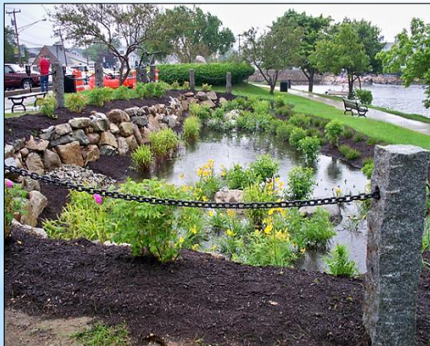
Bioretention basin at Water Street in Plymouth Center, Massachusetts. https://capecodgreenguide.wordpress.com/bio-retention/
