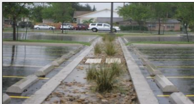
Bio-retention (McAllen, LRGV TX)
