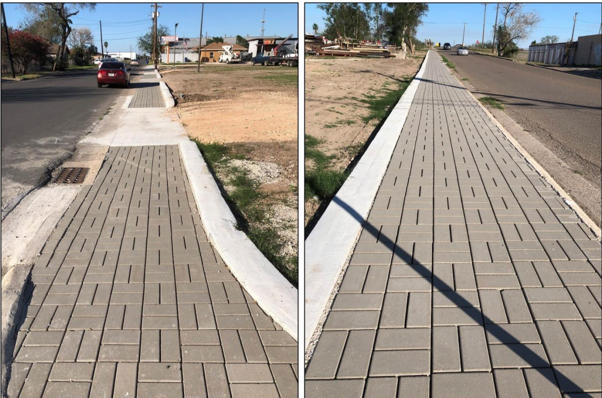
Figure 20. The two sides of the Permeable pavement after the construction
