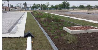
Bio-swale, (Brownsville, LRGV TX)
