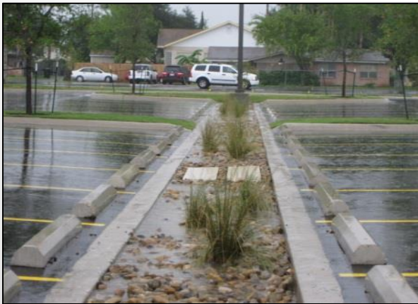
Bioretention (McAllen, LRGV TX)
