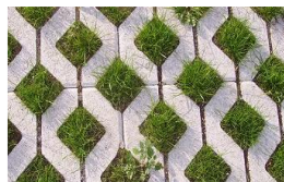
Permeable paving allows stormwater to drain into the soil rather than flow into drainage systems. Source: Wikipedia
