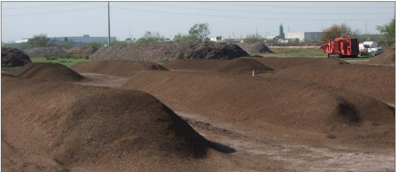
McAllen Composting Facility
