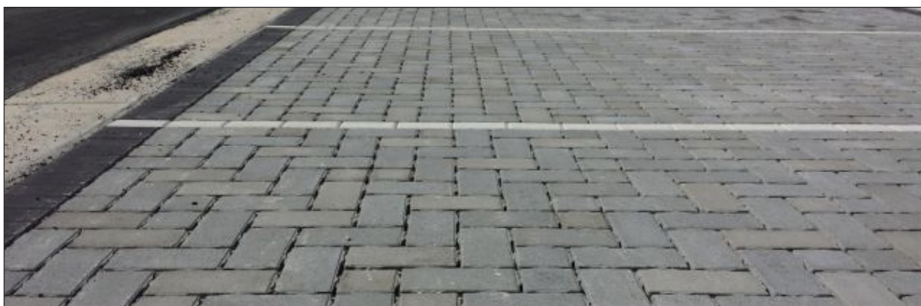
Example of pervious pavement
