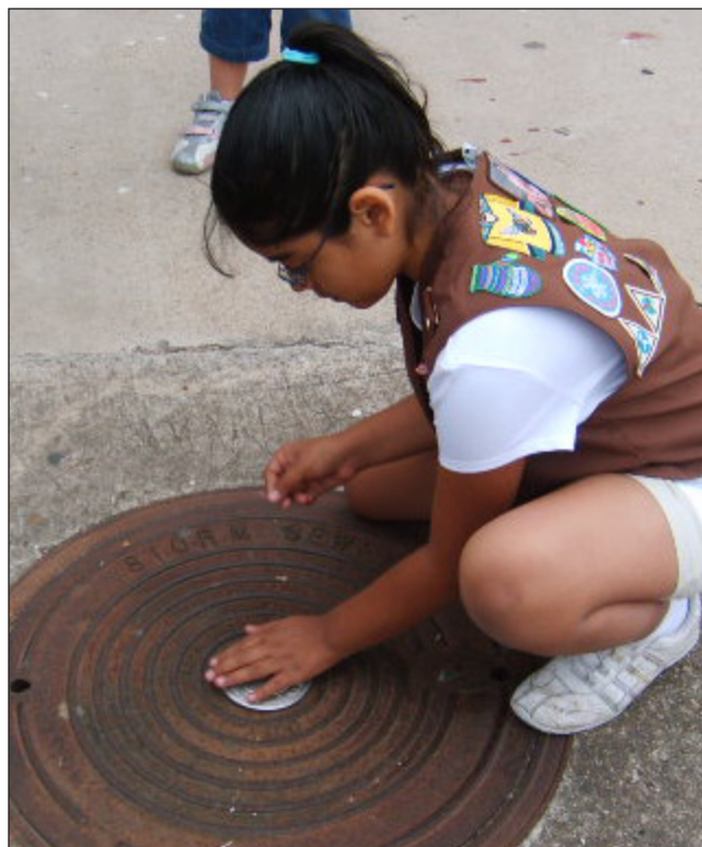
Brownie troop member installing storm drain marker
