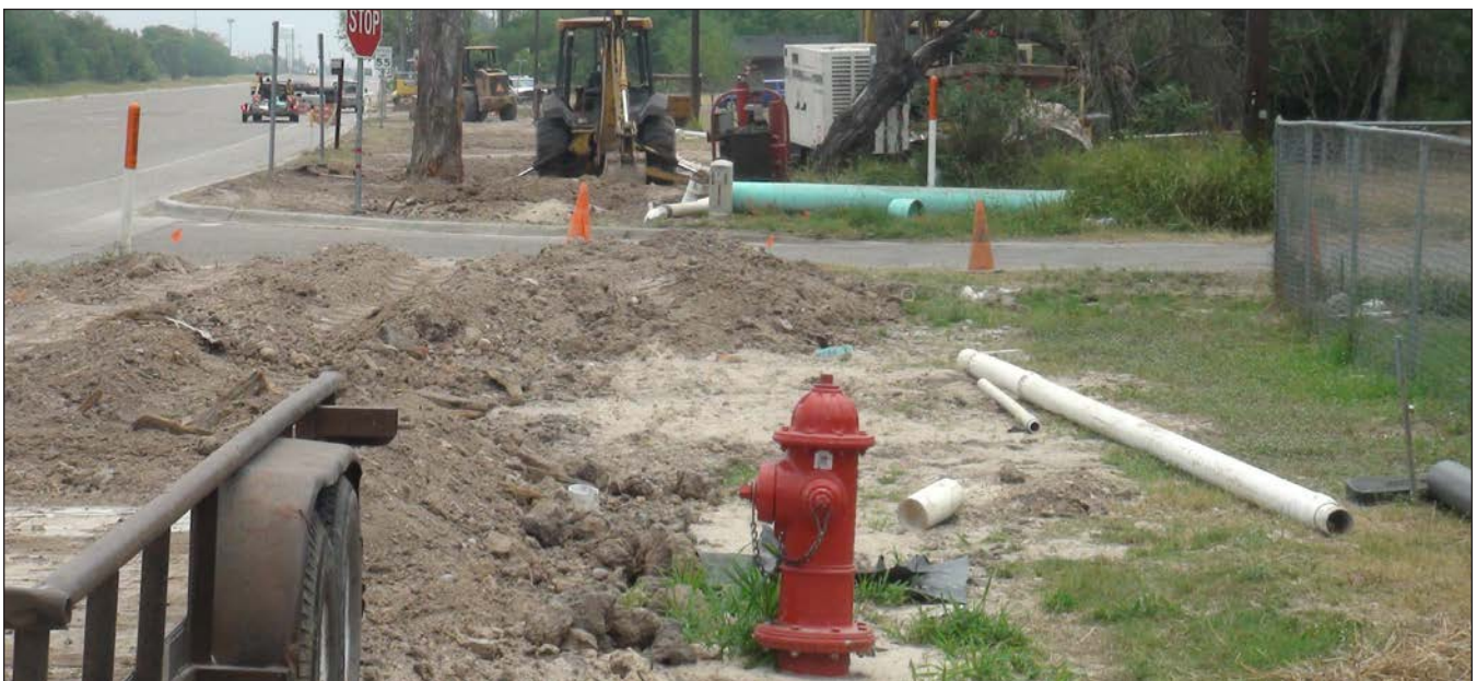
Installing potable water and wastewater infrastructure to colonia residents in La Feria, TX
