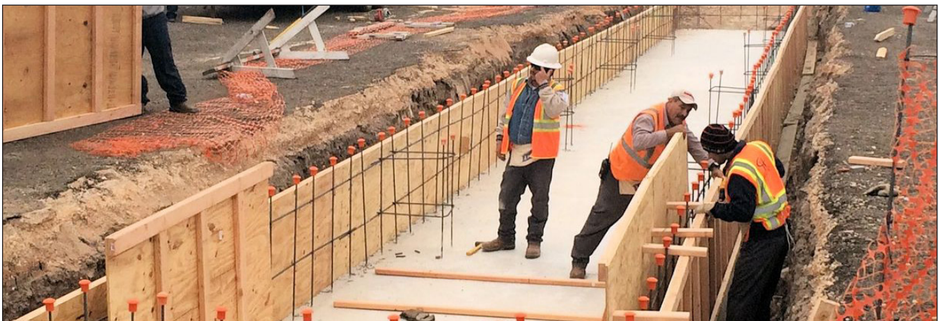
Construction of a bioretention basin at Ramsey Park, parking lot to collect and treat stormwater runoff
