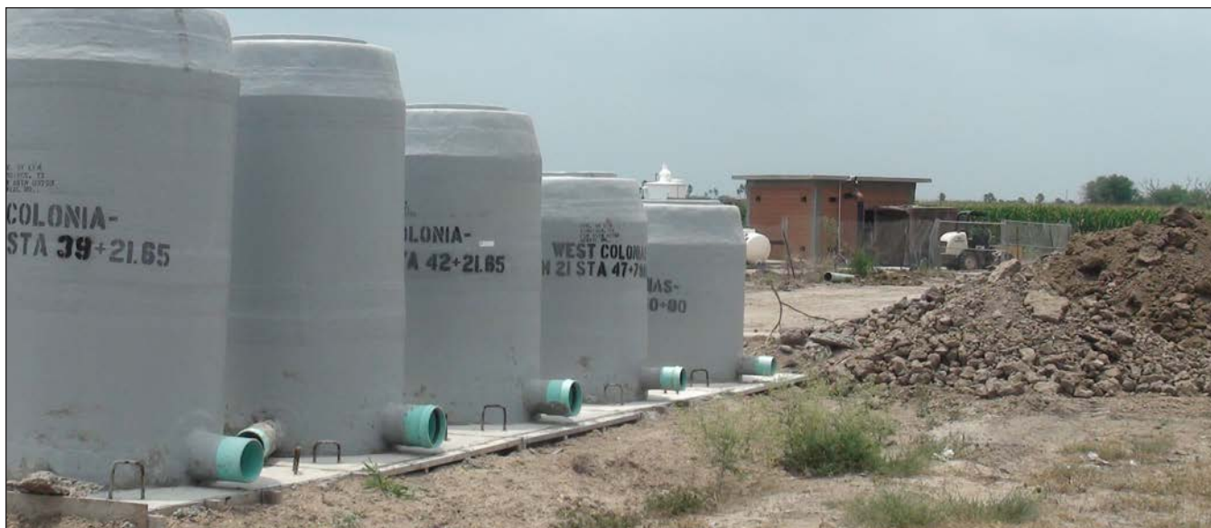
Sanitary sewer manholes to be installed with new lift station in the background, in La Feria TX
