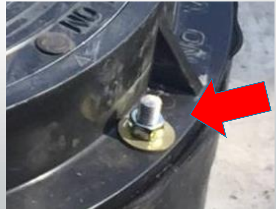
CAPs Frame Allows Seat for Nut & Washer
