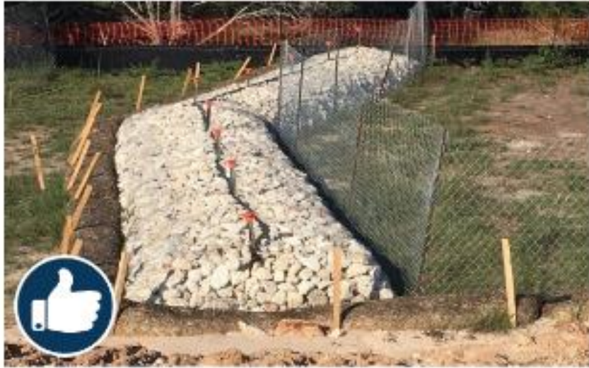
Properly installed check dam using a rock filter dam.
