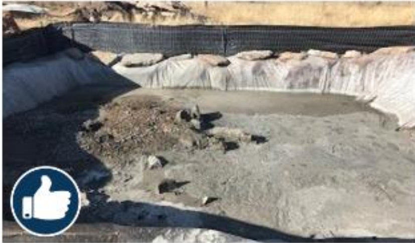
Designated washout area is fully contained.
