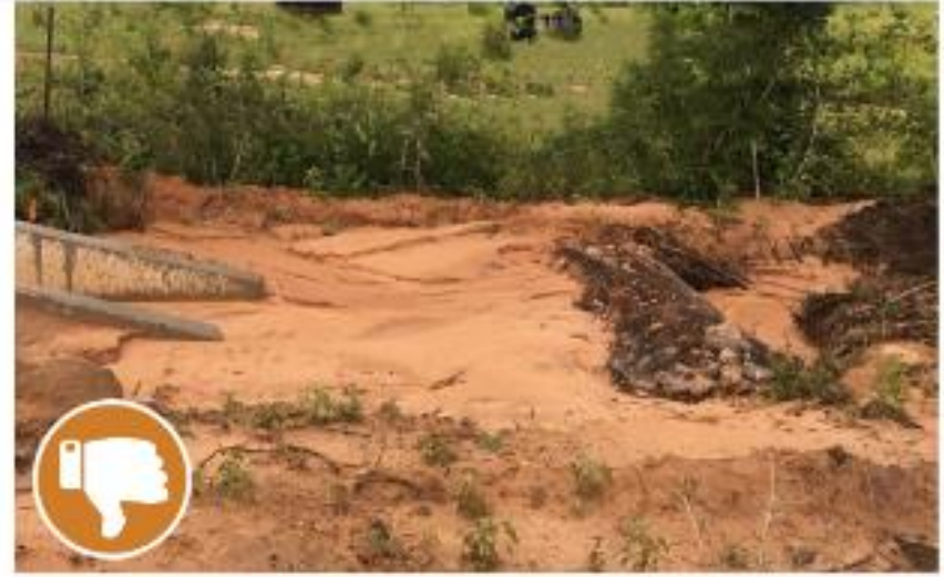
Failing BMP – dam is filled to capacity and in need of maintenance. The check dam should cover the entire length of the drainage. Silt and debris should be removed from the dam on a regular basis.
