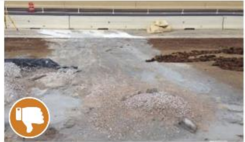
Washout area does not have proper containment which led to washout on the road. Post signs clearly labeling the washout location. BMPs surrounding the area should be maintained and managed and BMPs to prevent offsite tracking and runoff should be in place.
