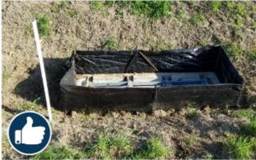
Properly installed inlet protection - fabric properly toed in, stakes are secure, adequate overlapping of fabric.
