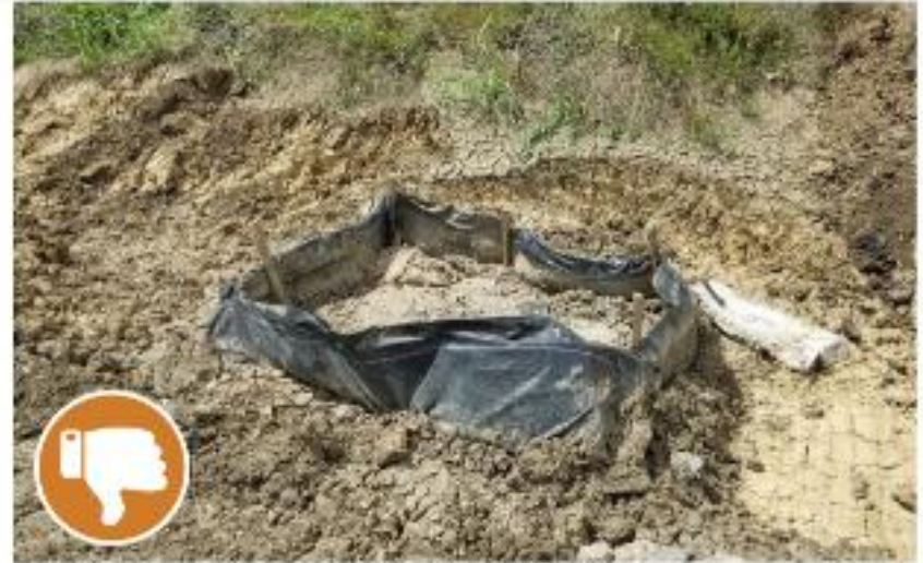
Failing BMP - inlet device has not been properly maintained. It is overwhelmed by sediment and is collapsing.
